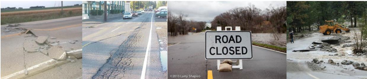
**Figure 1. Examples of pavement failure (l to r): Pavement buckling from high temperatures; fatigue cracking and rutting on an asphalt concrete pavement; road closure due to pavement inundation during a flood event; and pavement washout from a flood event.**
